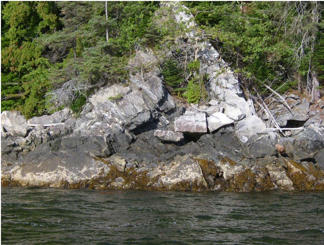
Photo 3-1 Rock Wall and Ramp, Sheltered
